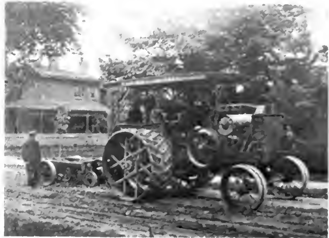
Fig. 8.—Scarifier operated by Traction Engine.
